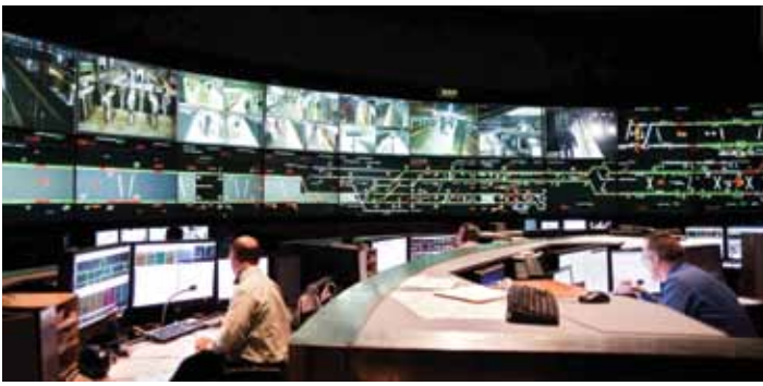
▲ Massachusetts Bay Transportation Authority, Boston, MA
